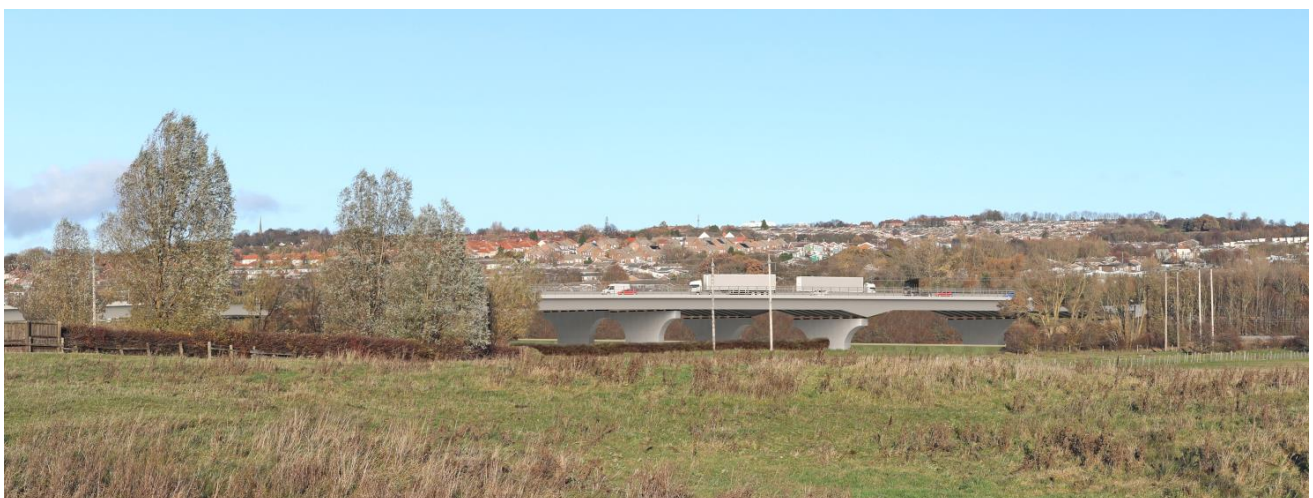
Figure 8 - Photomontage of north-east views from Lamesley Road (representing residential properties and visitors to St Andrew's Church) - Viaduct option
