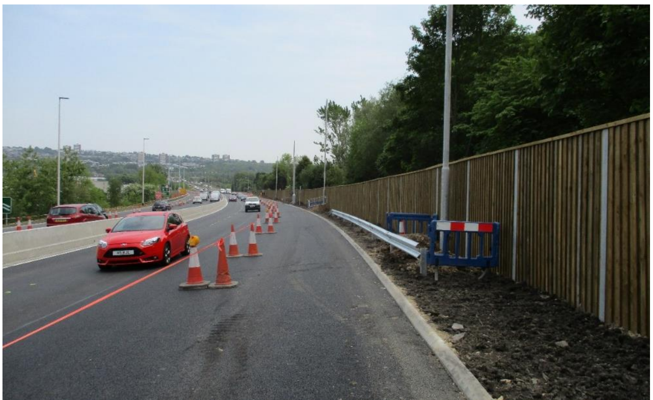
Figure 11 - Existing Noise Barrier at along Lady Park adjacent to the A1
